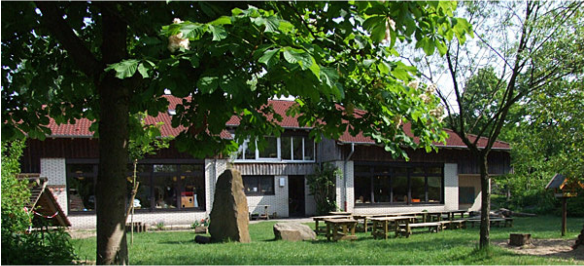
Ev. Kindergarten in Kattenvenne
